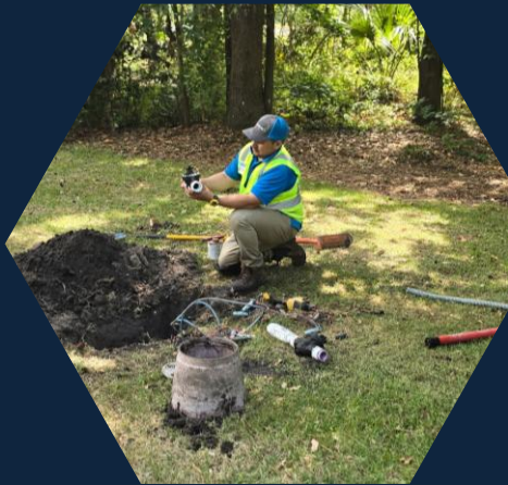
Irrigation Valve Replacement
